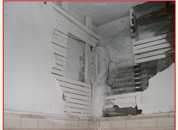
Fifty years of dampness has caused failing plaster and concrete throughout the basement.
